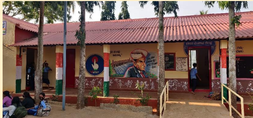
Photo 13: Painting work at the school
